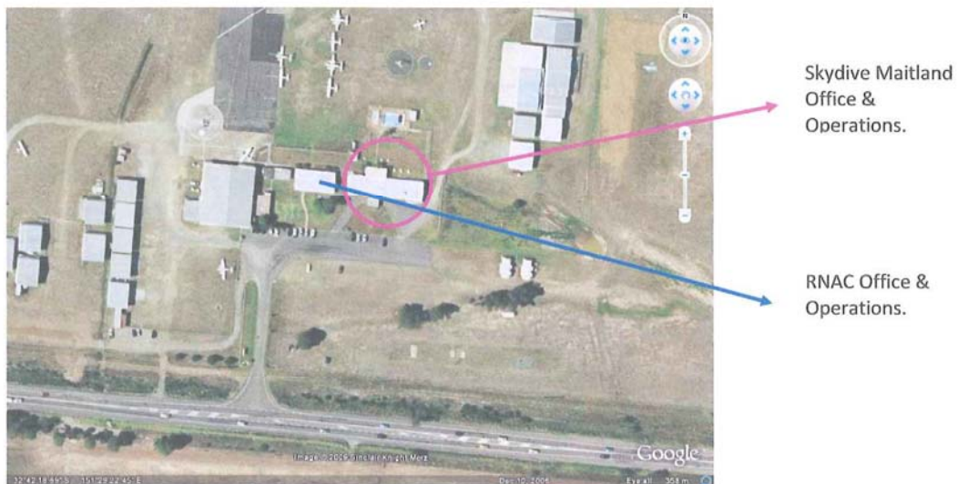
Figure 1~ Aerial photograph (Google Earth) shows the building (circled in pink) which Skydive Maitland will conduct business.
